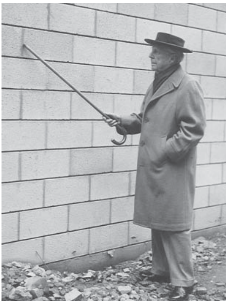
Frank Lloyd Wright examines the curved, cinder block retaining walls.
